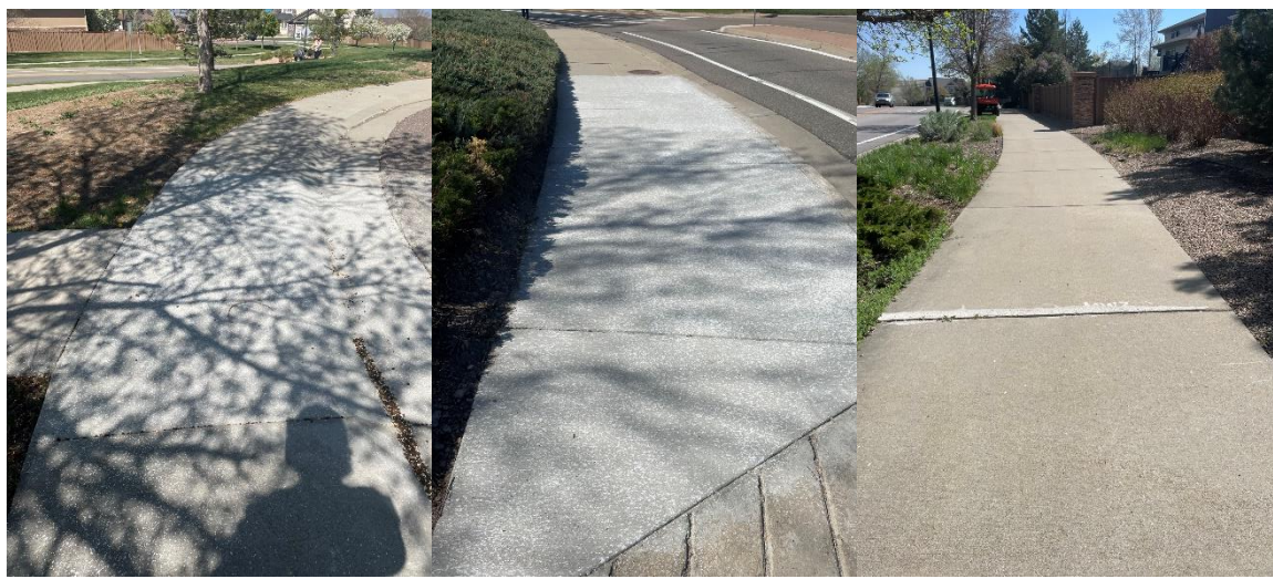
MW1, MW2, AND MW3 COMPLETE
